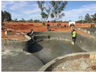
There is still a fair way to go before the pool can actually be swum in, but we are getting there. Hopefully, over the next few months the splash pad base will be poured, along with rendering and finishing of the base structure taking place.
