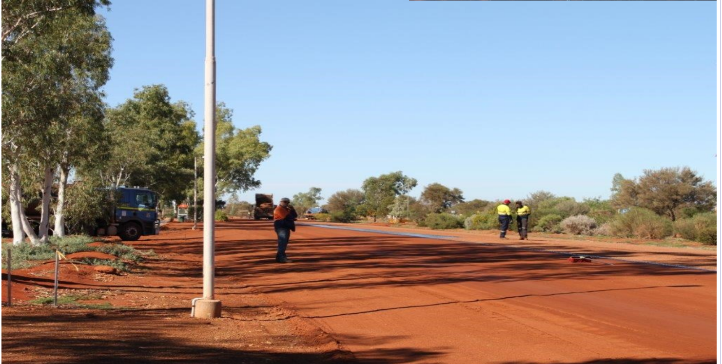
You can't take, 'the stand around doing nothing,' out of a good shire worker. Brian Wundenberg Works Supervisor, keeping an eye on the sealing.
