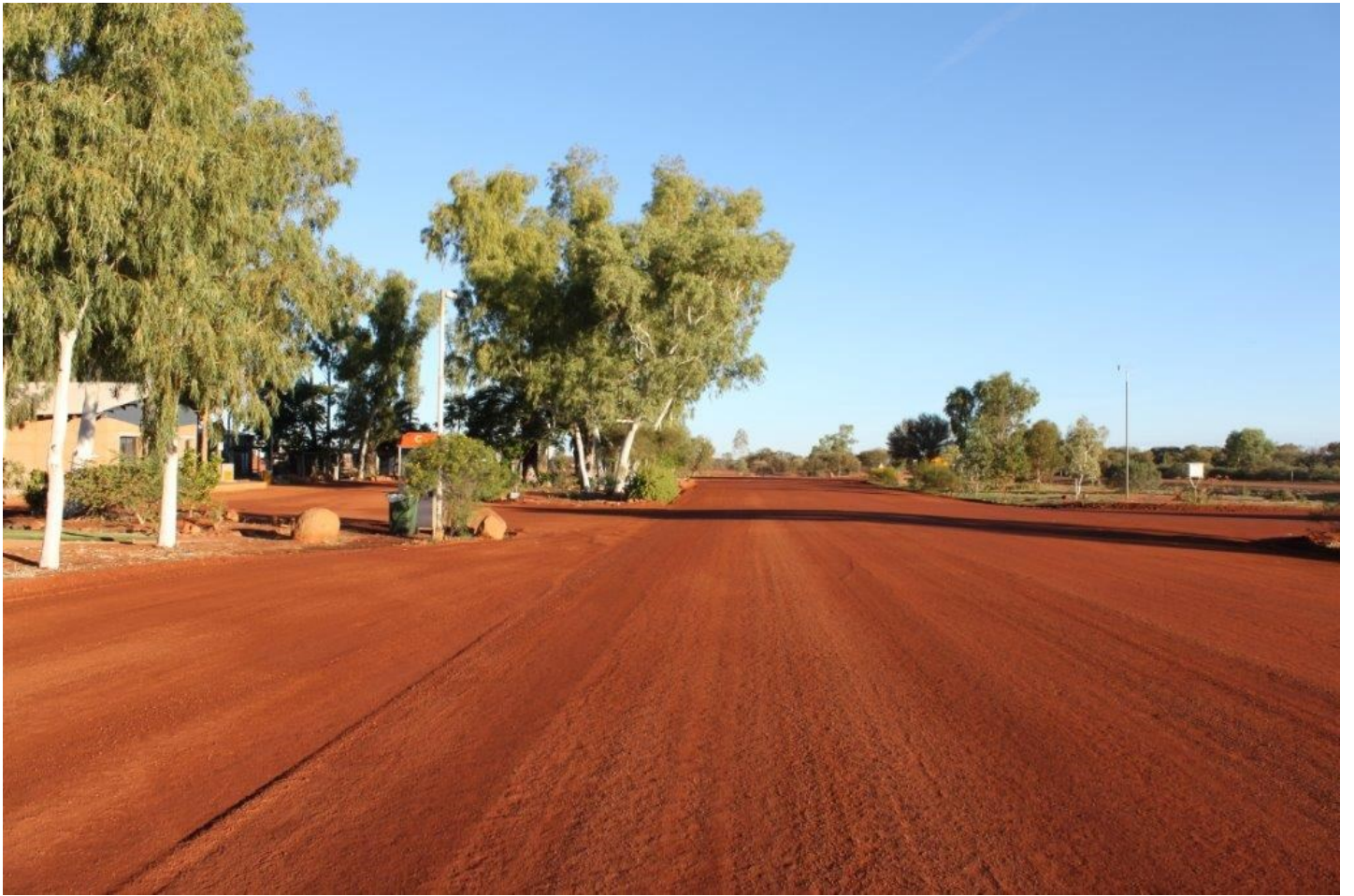
Final trim done and ready for the bitumen
